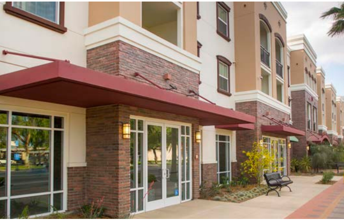
Example: Awnings are an example of functional ornamentation, providing both shade and articulation.
