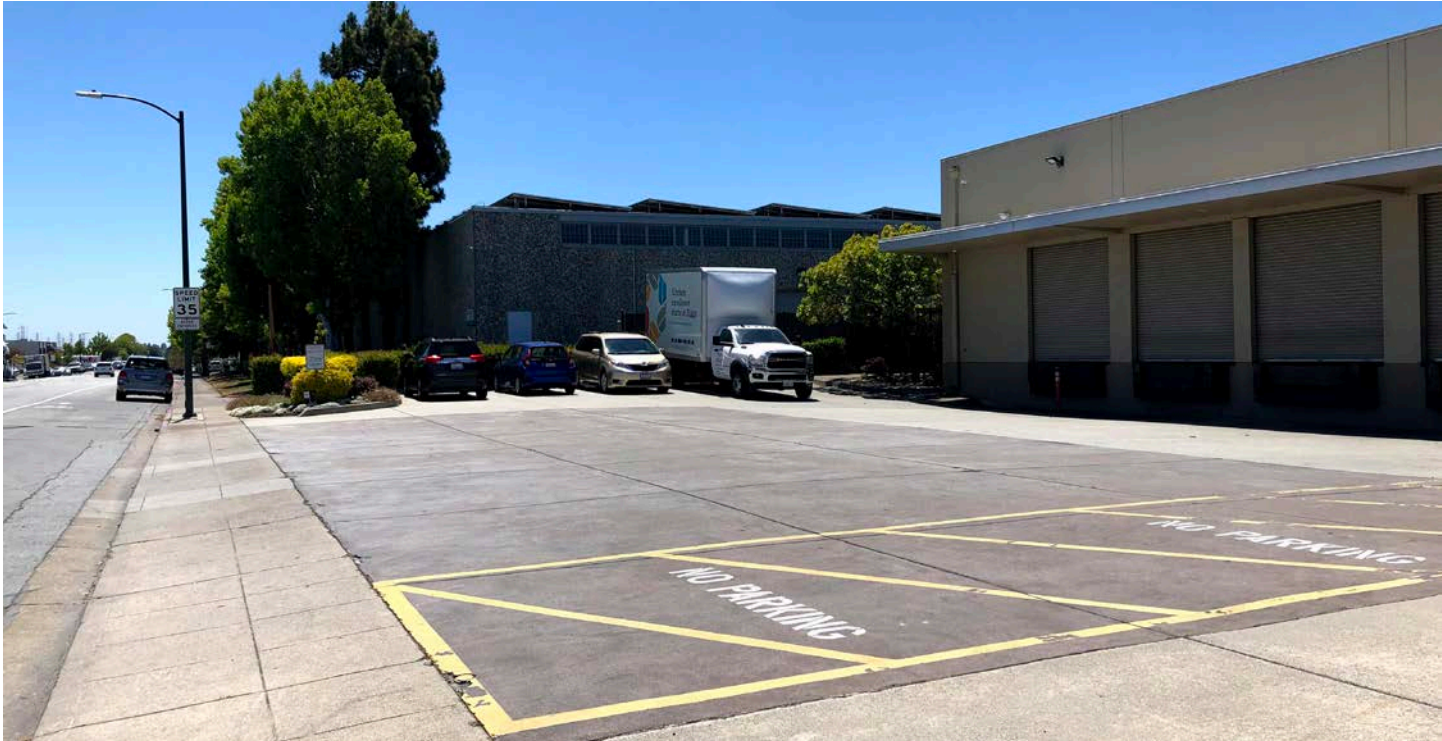
1755 Rollins Road – long curb cut through sidewalk for trucks and loading.
