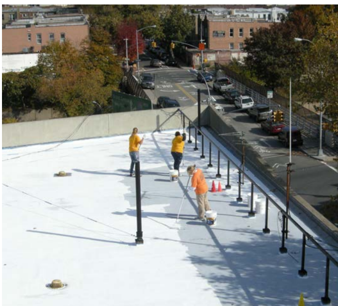
Example: Cool Roof Installation
