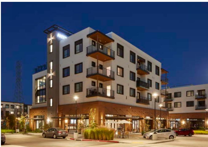
Example: Mixed-use development with non-residential uses on the ground floor, and dwelling units on upper stories.
