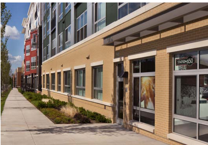
Example: Horizontal banding and massing breaks distinguish various uses within the same structure.
