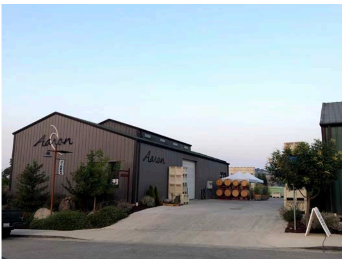
Example: Overall massing of development reduced by breaking building into smaller sections.
