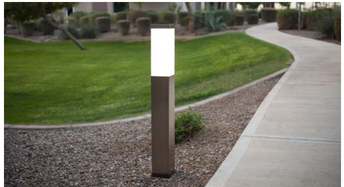
Example: Lighted Bollards provide illumination along pedestrian walkways and at increase light levels at building entries.
