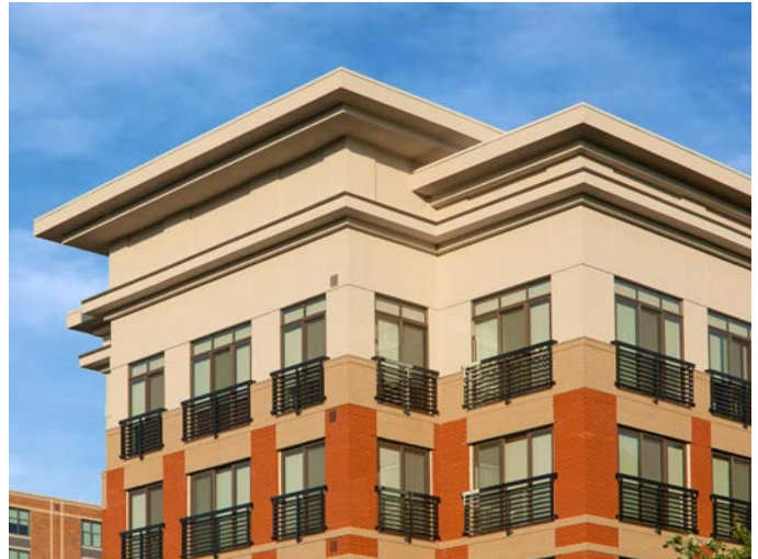
Example: Cornice elements are well-integrated with the building's overall design in both form and materials.
