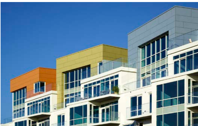
Example: Vertical roof plane breaks divide the vertical massing and rooflines into sections.
