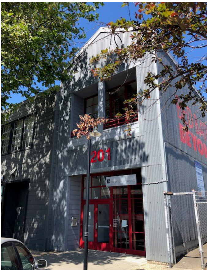
Example: Building massing concentrated along the street, with clearly marked and recessed pedestrian entry.
