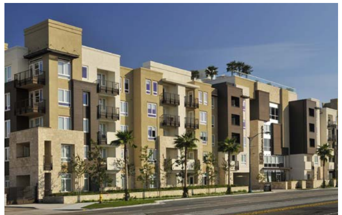
Example: Five-story podium structure includes parking on lower stories with dwelling units located above.
